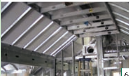
1) Front view of completed house. 2) Exterior side walls are erected. 3) All Roof Panels are installed and secured, gabled windows ready for finishing. 4) White siding is applied with screws directly to the Snap-N-Lock™ Panels. Soffits become unnecessary because of the clean white underside of the metal panels. 5) Close-up of floor trusses. 6) Close-up of upper-level steel interior framing and furring channels. 7) Side view of completed home.
